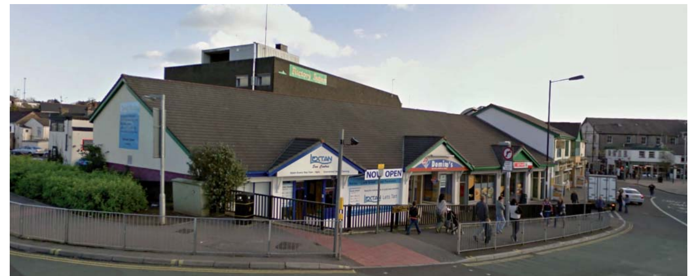
View of potential Market Street/Quarella Road/Derwen Road from Quarella Road/A4061
